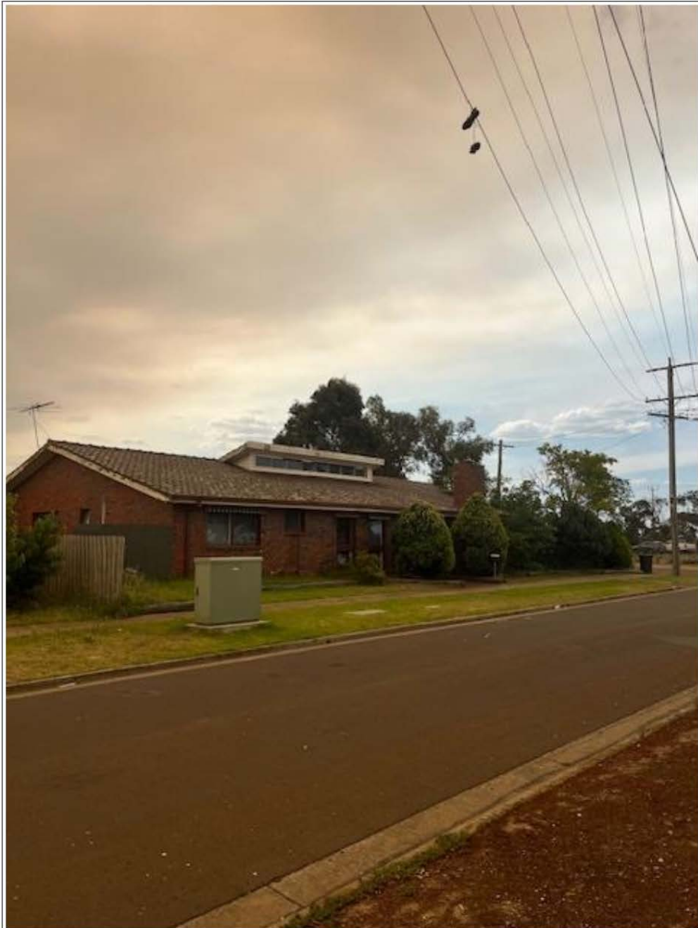
Leonid Drive Frontage of Subject Site – 20 December 2024
