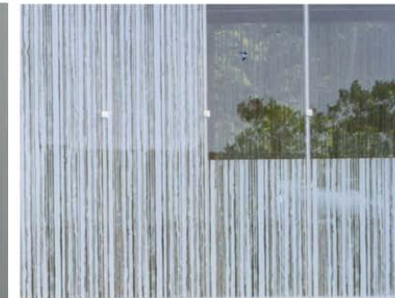
screen print pattern glass to selected spandrel panels
