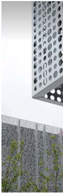
perforated metal to sunshades, balustrades and main canopy
