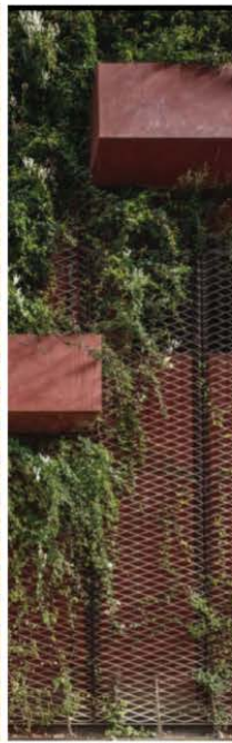
steel and timber framed landscape trellis columns
