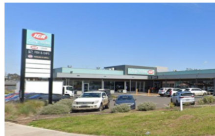
Figure 44. IGA City Vista Court Plumpton
