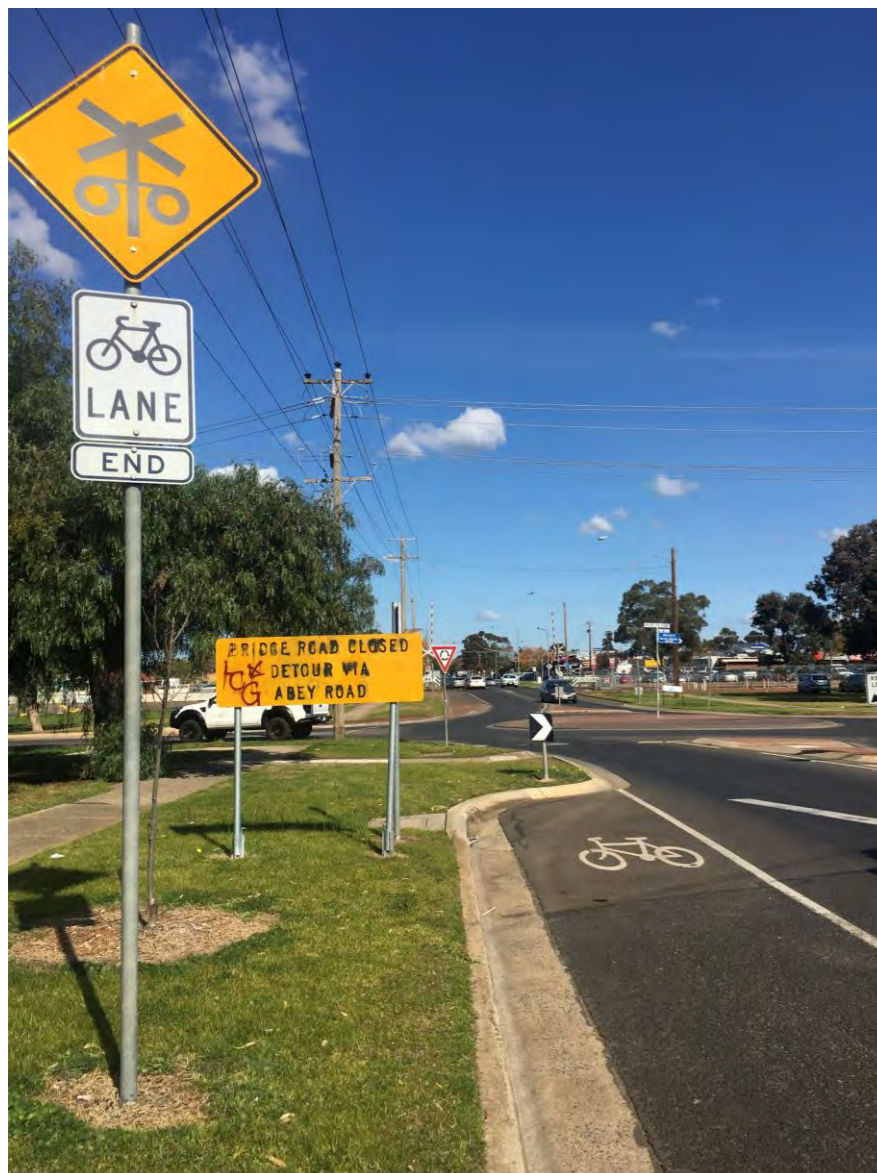
Figure 36: Path ends before the roundabout and cyclist is not supported through the intersection
