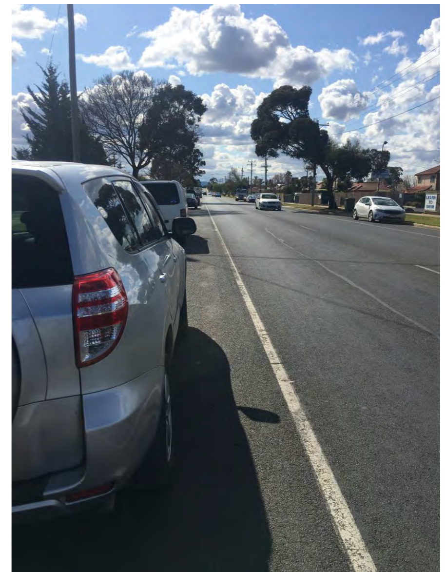
Figure 38: Path is very narrow and places riders within the 'dooring' zone on a 60km/h street
