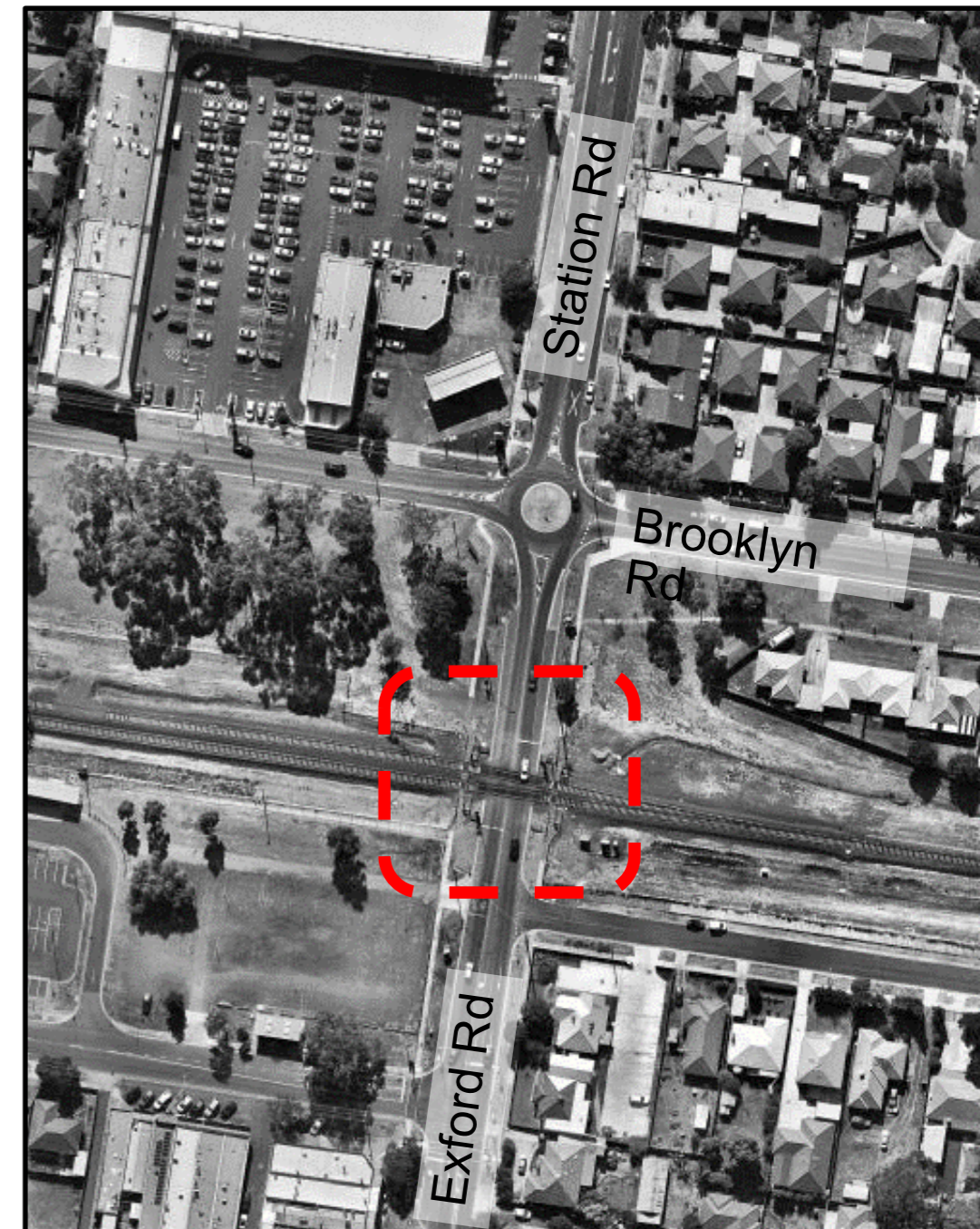
Figure 20: Exford Road level crossing Source: Nearmap
