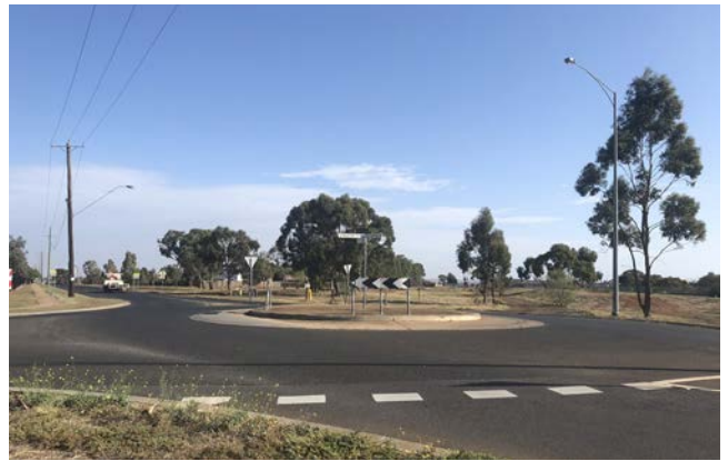
Fig. 44 Coburns Road and Staughton Street intersection
