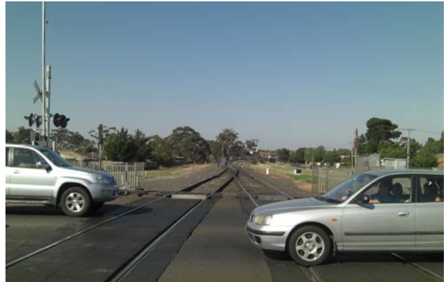
Fig. 26 Current at-grade rail crossing
