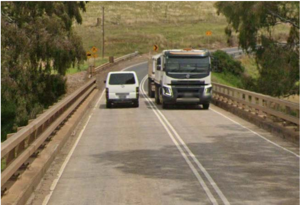
Figure 3 – Exford Road Bridge looking west. Google Street View February 2021
