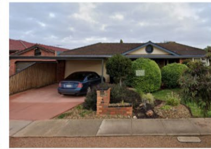
NO. 10 GALILEE BLD (AJJOINING SITE) SINGLE STOREY BRICK HOUSE TILE ROOF
