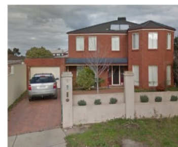
NO. 7 COMIC COURT (ADJACENT SITE) DOUBLE STOREY BRICK HOUSE TILE ROOF
