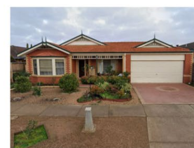
NO. 12 GALILEE BLD (ADJACENT SITE) SINGLE STOREY BRICK HOUSE TILE ROOF
