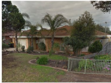
NO. 5 COMIC COURT (SUBJECT SITE) SINGLE STOREY BRICK HOUSE TILE ROOF
