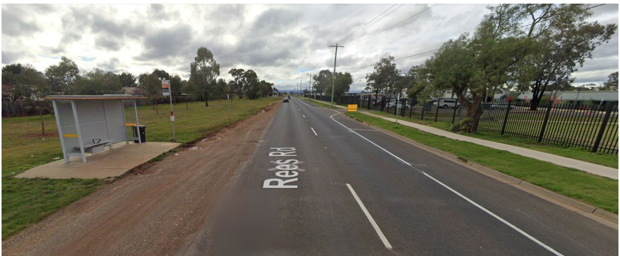
Figure 2 Rees Road looking north
