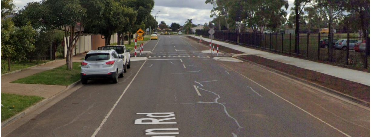
Figure 3 Wilson Road looking west
