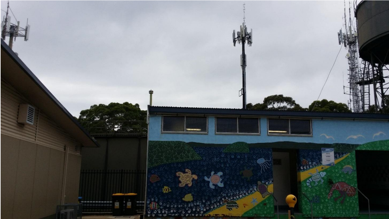
Figure 5 - Two monopoles and a lattice tower, all on the same site, within metres of one another
