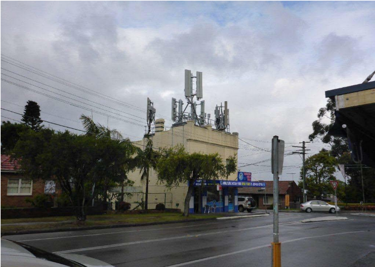
Figure 6 - An obtrusive and overcrowded rooftop
