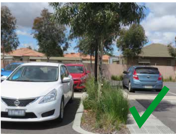
Figures 65 and 66 - Passive drainage into landscape areas improves soil moisture and landscape health
