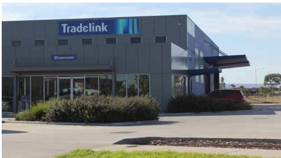
Figure 32 - Building with appropriate height office closest to street frontage and larger main building tapering up away from the street frontage and including windows to articulate the facade
