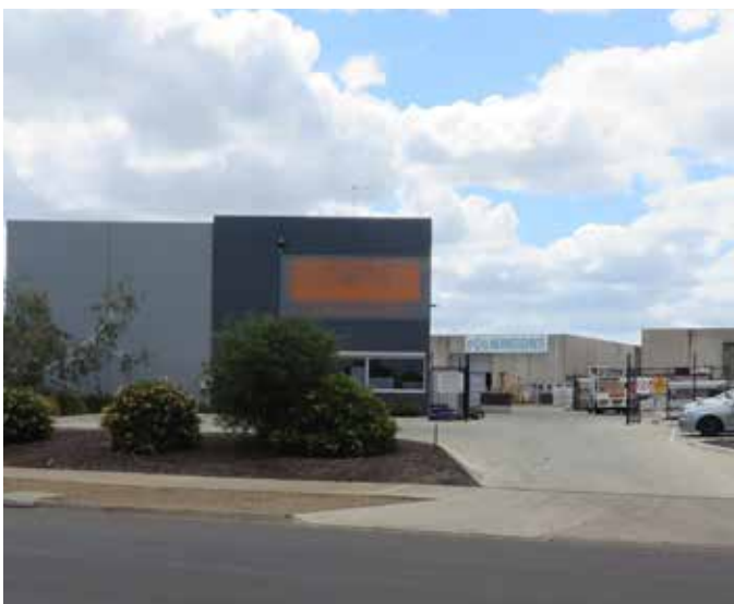
Figure 12 and 14 - Irregular shaped allotments often result in a poor building address to the street due to design requirements such as access and parking
