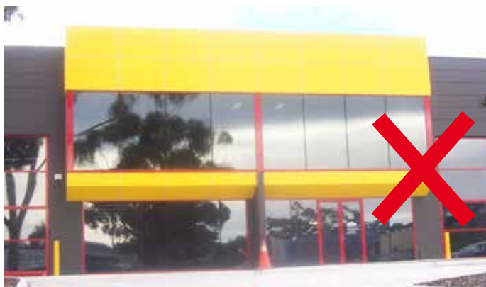
Figure 52 - Use of bright colours in large portions is likely to render an overly synthetic building appearance
