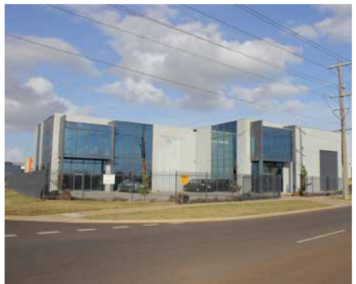
Figure 14 - Orientate lots to the higher order street to promote better activation and visual interest on main streets
