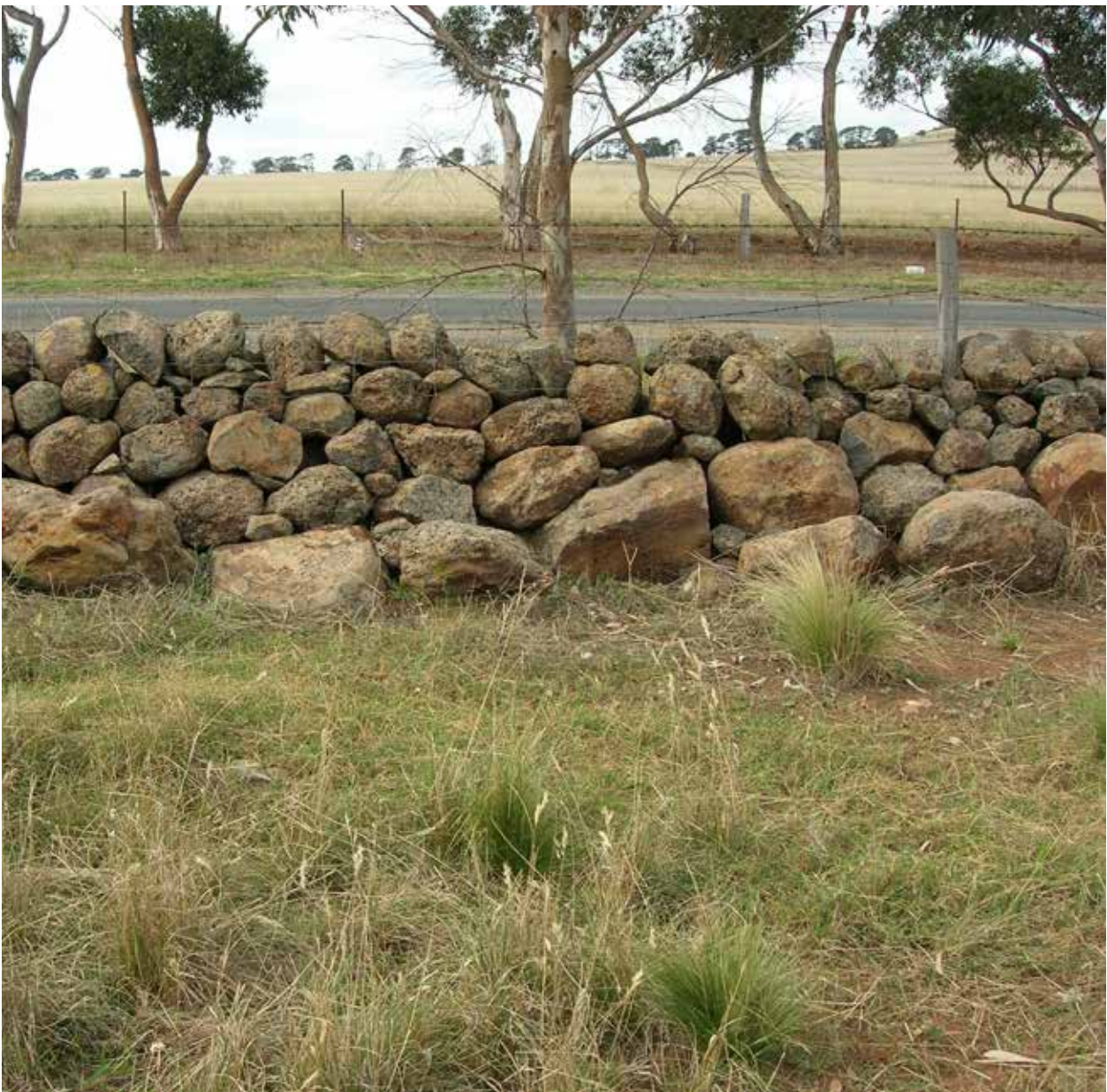
DRY STONE WALLS.
