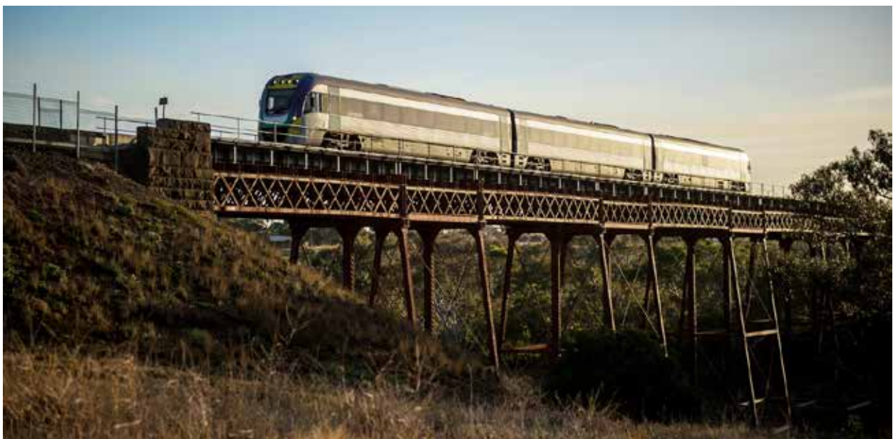
A VLINE RAILWAY SERVICE PASSES OVER THE MELTON WEIR VIADUCT.
