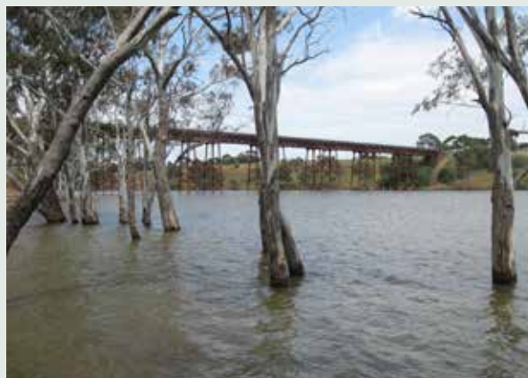
MELBOURNE-BALLARAT RAILWAY LINE CROSSING OF THE MELTON WEIR.
