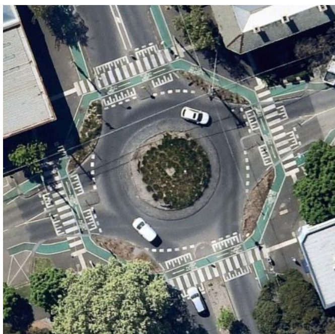
Figure 4 Protected roundabout, South Melbourne
