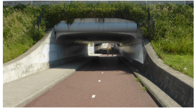
Figure 86 Walking and cycling underpass, The Netherlands
