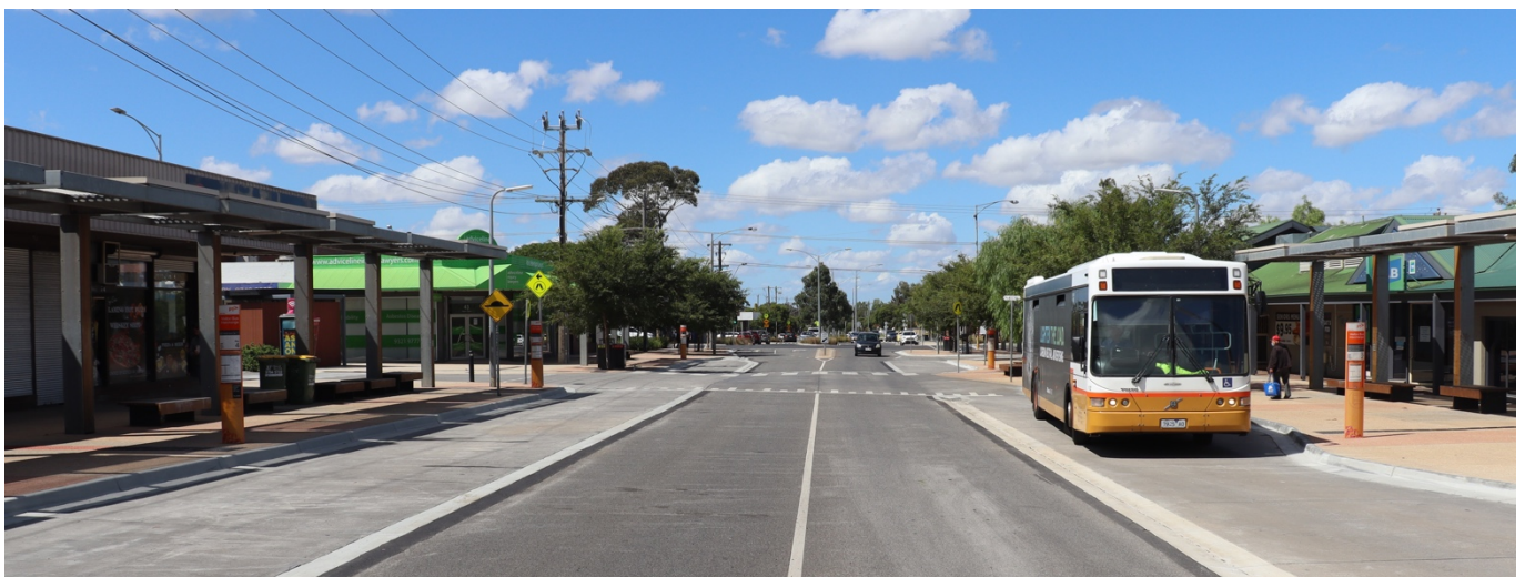
Figure 90 Melton Bus Interchange in Palmerston St
