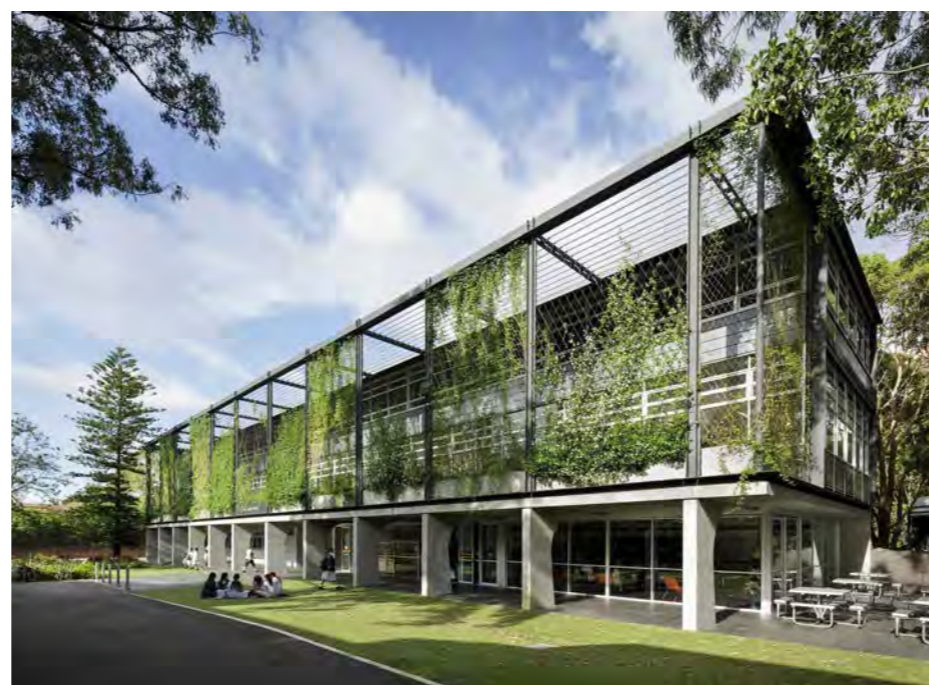
Example of vertical vegetation facade system which will lower the ambient temperature of the centre
