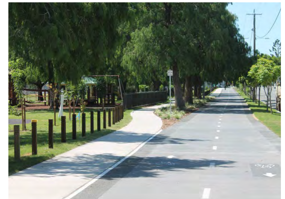
Bi-directional cycling path, separated from both the pedestrian walkway and the road carriageway
