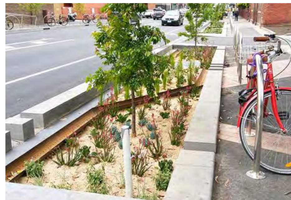
Example of an on-street rain garden which assists with stormwater attenuation and adds amenity to the streetscape
