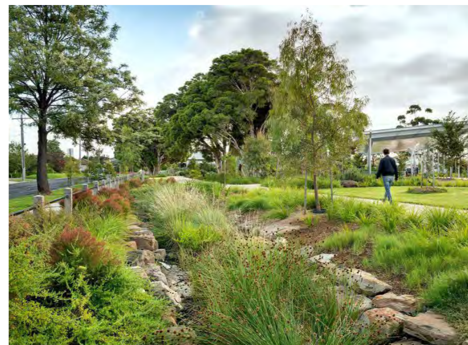
Example of a central stormwater bioswale allowing for water to be filtered prior to entering the stormwater system
