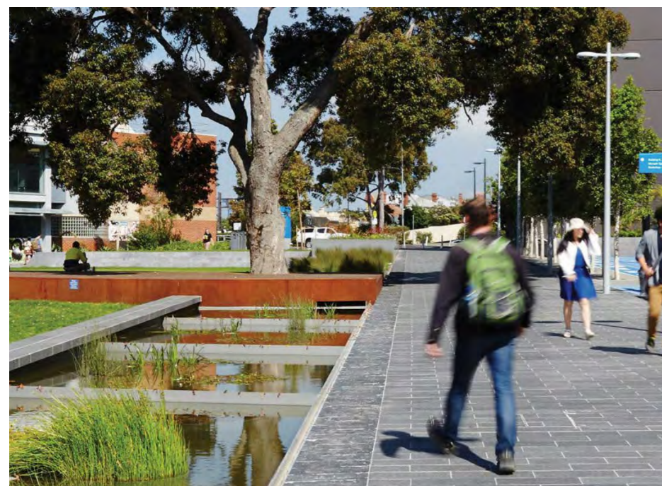
Example of stormwater storage and filtration adding to the amenity of the public realm
