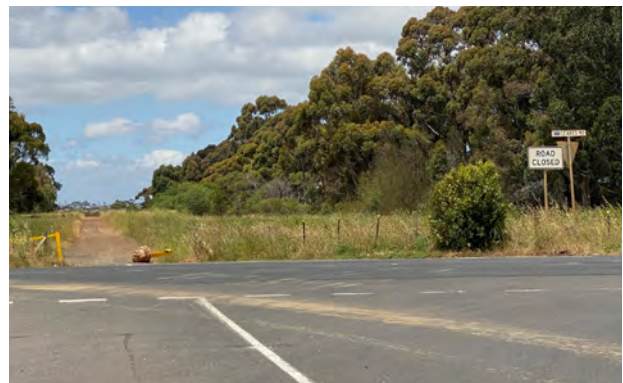
Beattys Road intersection view east
