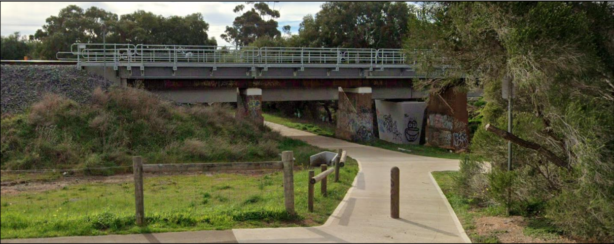
Figure 14: Existing Rail Underpass – West Side of Toolern Creek
