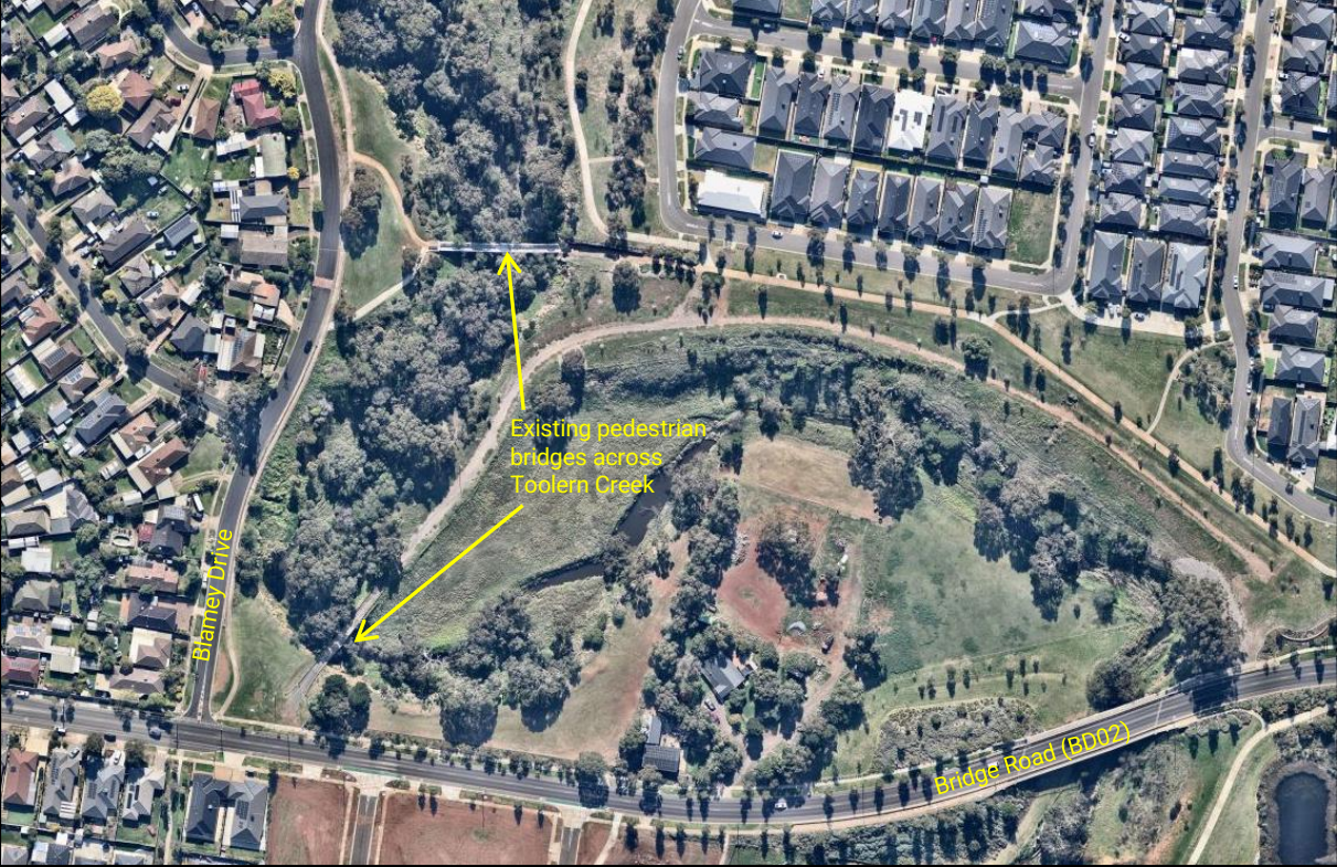
Figure 13: Existing Pedestrian Bridges Across Toolern Creek (not in DCP)
