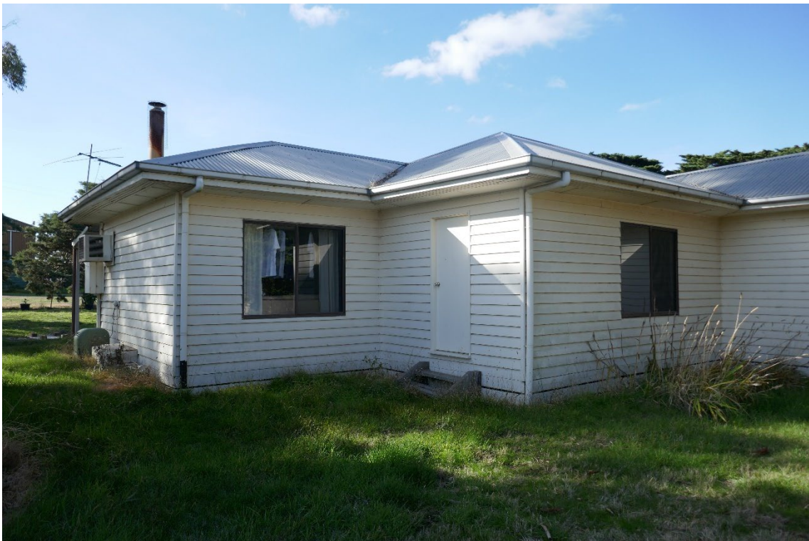
Figure 10 No. 740-794 Mount Aitken Road, south elevation (part) as modified: compare with Figure 11
