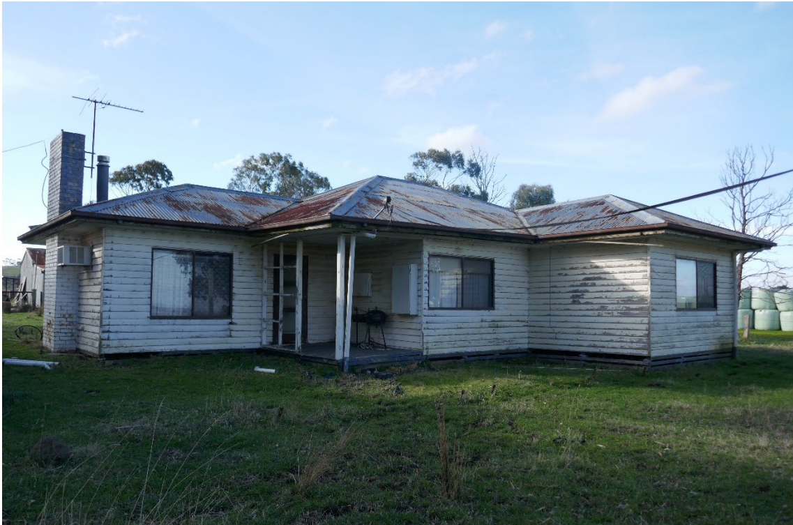
Figure 11 No. 796-830 Mount Aitken Road, south elevation
