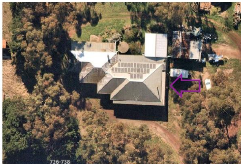
Figure 12 Aerial view of 726-738 Mount Aitken Road: the large addition is indicated Source: Nearmap (accessed 26 May 2023)
