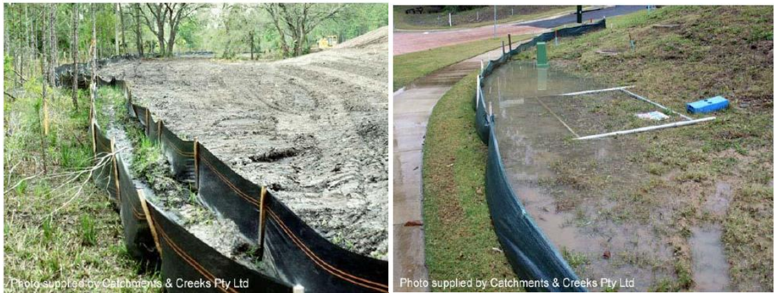
Plate 1: Photo of sediment fences installed correctly
