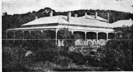
VIEW OF HOMESTEAD
