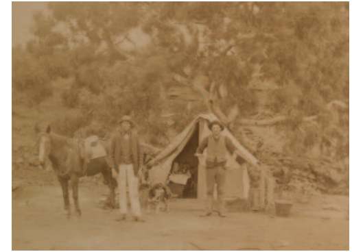
Workmen engaged in the construction of the Melton railway viaduct over the Werribee River, c. 1884. Campsites for the workers were set up nearby.
