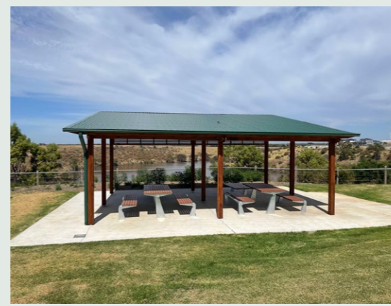
Double skillion roof shelter as installed in Weir Views
