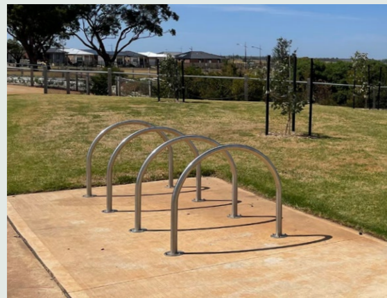
Council standard bicycle hoops as installed in Weir Views
