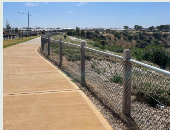
Fencing as installed in Weir Views
