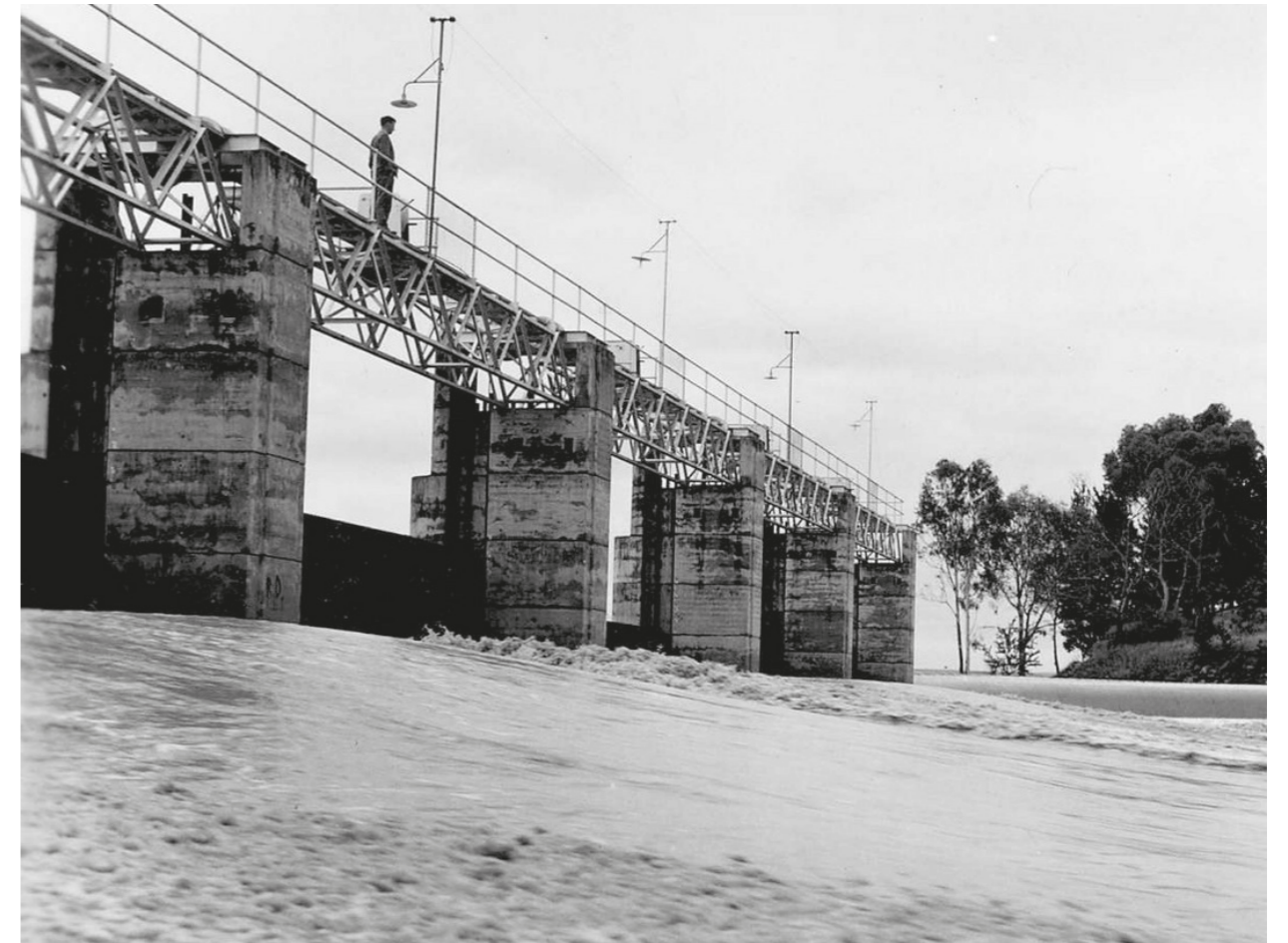
FIGURE 1.2: Construction of the Melton Dam. Source: State Library of Victoria, 1940's
