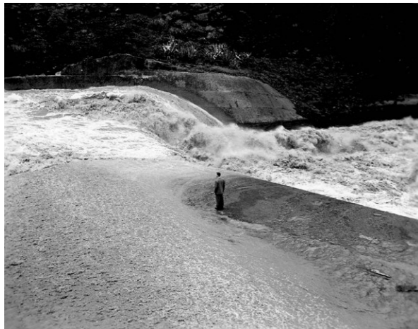
FIGURE 1.3: Melton spillway and regulator gates. Source: State Library of Victoria, 1954
