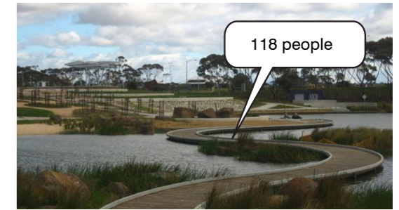
Water Crossing (Source: Melbourne Cairnlea Lake Boardwalk, Hassell)
