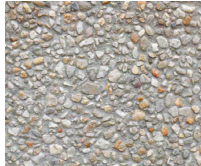
Exposed Aggregate Concrete
