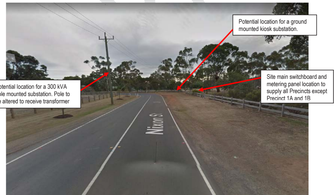
Fig 6 Potential substation sites, view looking north along Nixon Street from Reserve Road
