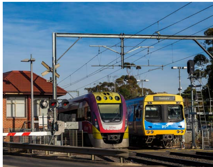
Electrification of rail line
