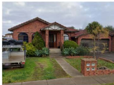
NO.8 GALILEE BLD (ADJACENT SITE) SINGLE STOREY BRICK HOUSE TILE ROOF
