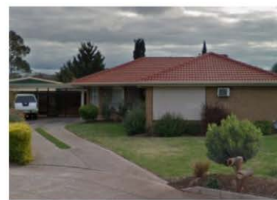
NO. 10 COMIC COURT (ADJACENT SITE) SINGLE STOREY BRICK HOUSE TILE ROOF
