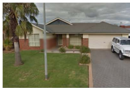
NO. 3 COMIC COURT (ADJACENT SITE) SINGLE STOREY BRICK HOUSE TILE ROOF
