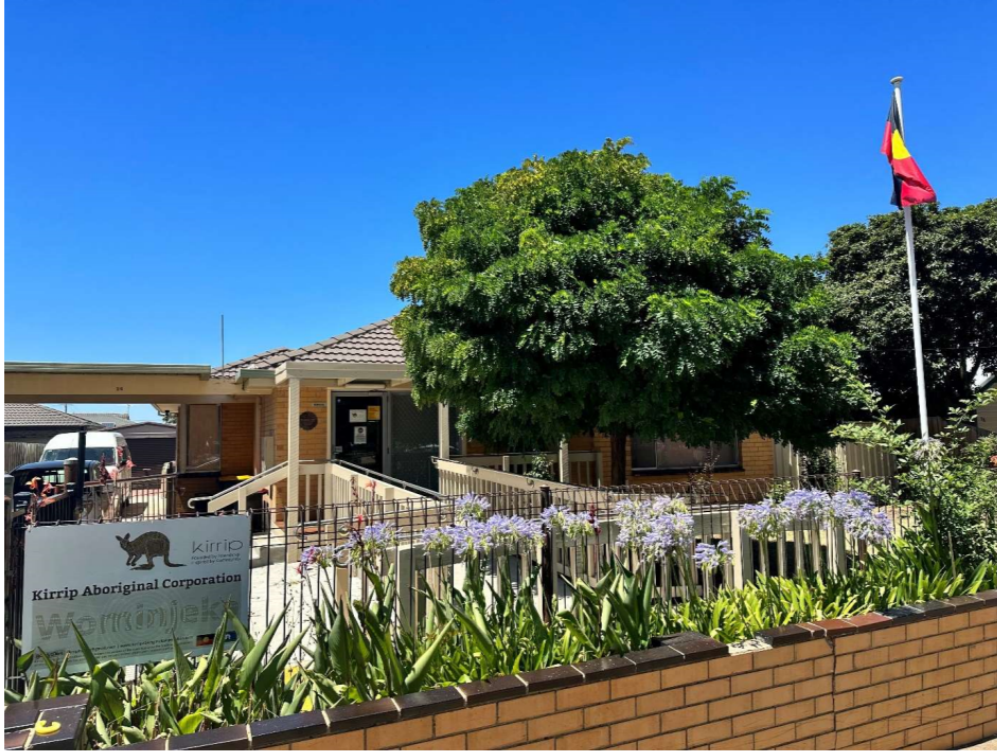
Figure 5: Photo of Kirrip’s main site – 26 Exford Rd, Melton South
