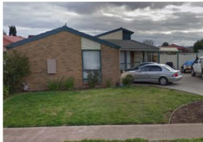
NO. 11 COMIC COURT (ADJACENT SITE) SINGLE STOREY BRICK HOUSE TILE ROOF
