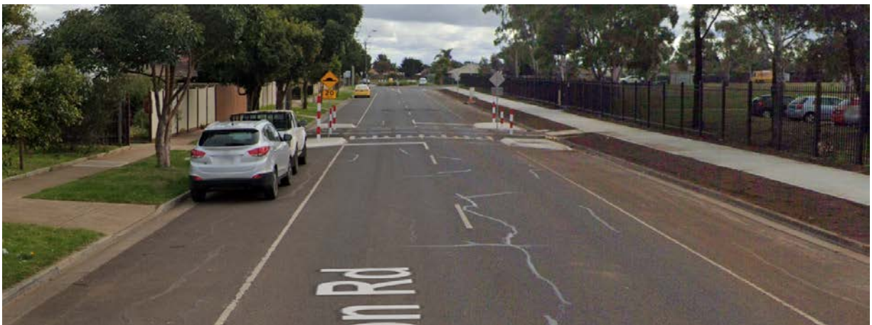
Figure 3 Wilson Road looking west
