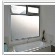
SELECTED FIXED AND AWNING OBSCURE GLAZING
