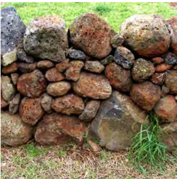
Dry Stone Wall
