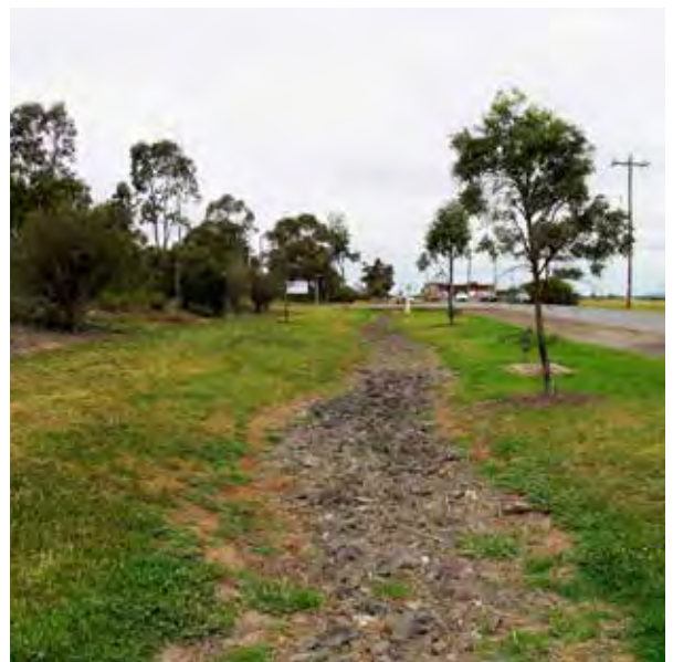
Existing Drainage along Arterial Roads
