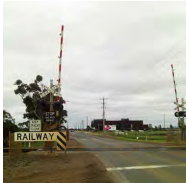
Railway Crossing (Ferris Rd)
