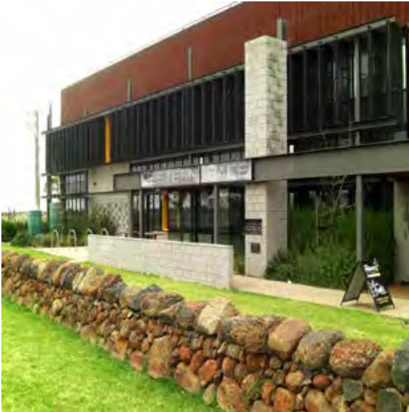
Western BACE (Business Accelerator and Centre of Excellence)
