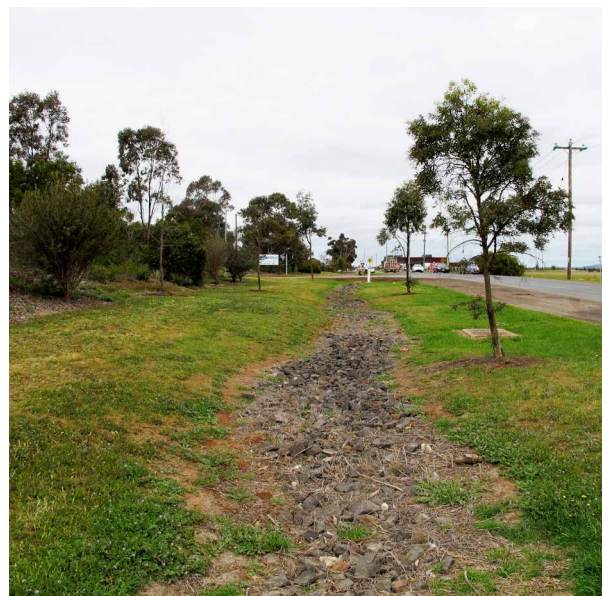
Existing Drainage along Arterial Roads
