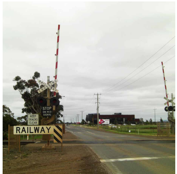
Railway Crossing (Ferris Rd)
