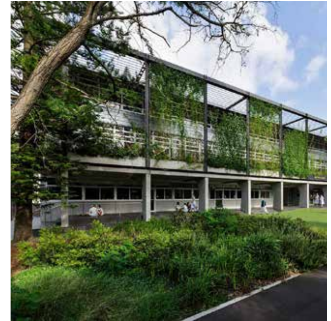
Image 27 Example of increased vegetation cover on building facades which will lower the ambient temperature of the centre
