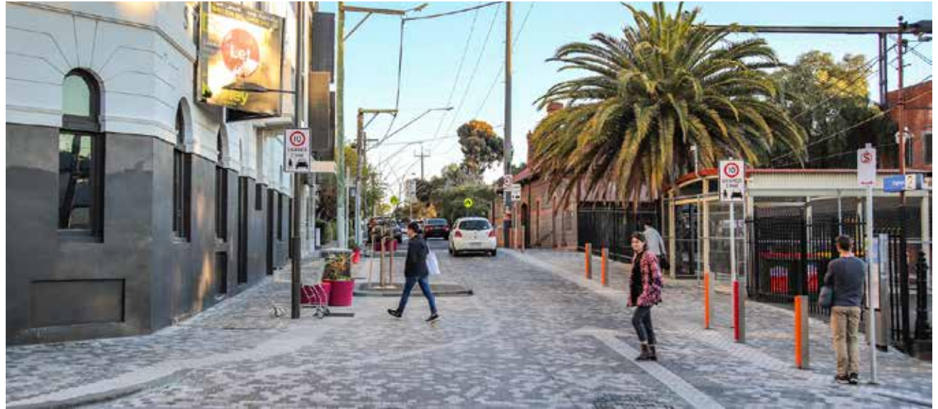
Image 11 Example of shared cycle and vehicle streets, with pavement details that enable slow vehicle speeds, and encourage movement
