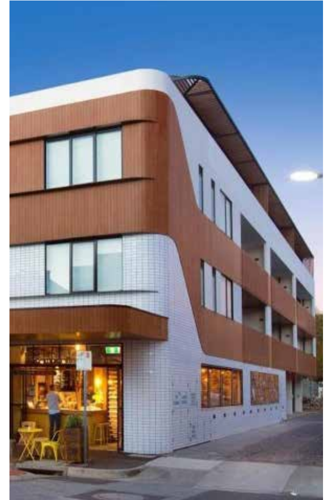
Image 23 Example of fine grain, texture rich architectural treatment on the ground floor
