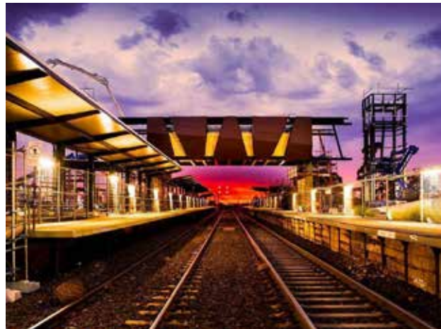
Image 8 Rockbank Station upgrade, under construction
