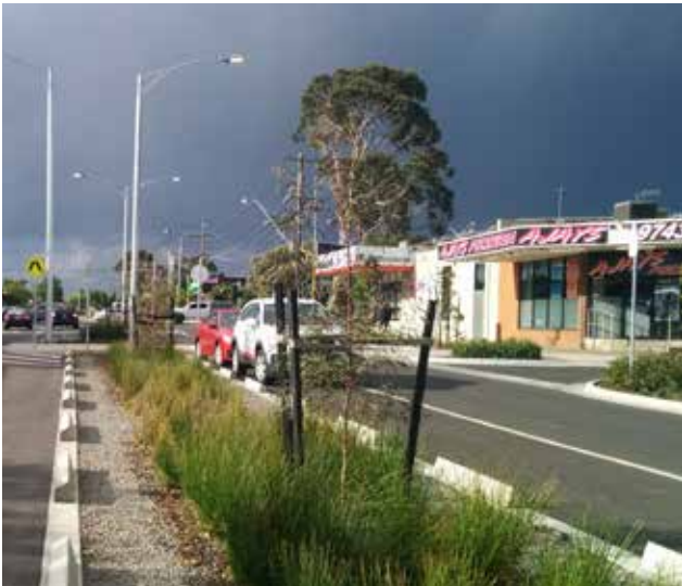
Image 30 Example of central swales allowing for water to be filtered and cleaned, prior to entering the stormwater system
