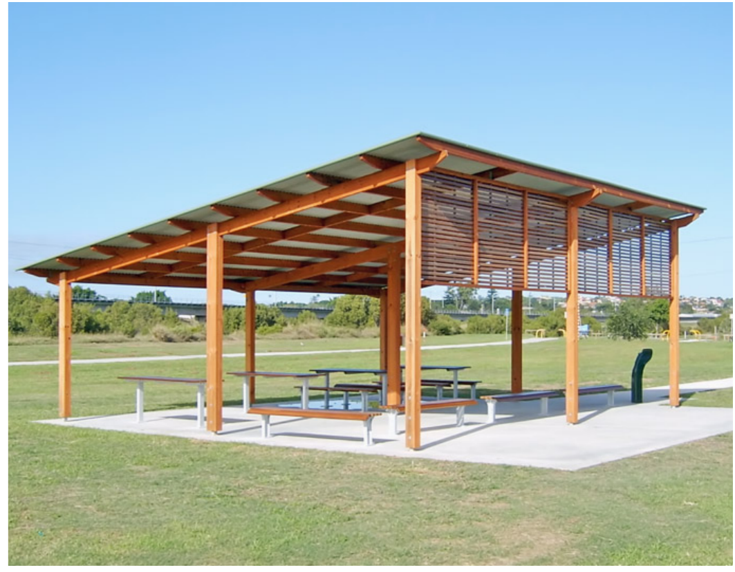
Generous picnic shelters with wheelchair accessible BBQs and table settings
