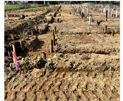
South Pavilion slab preparation
