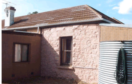
Figure 17 House - North elevation (west end)
