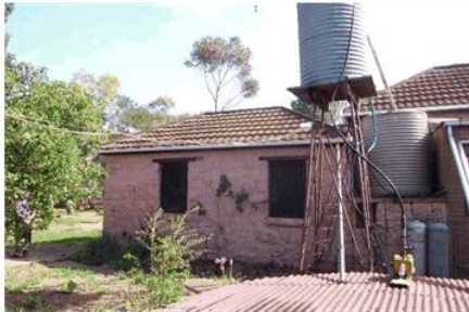
Figure 19 House - West elevation (north end)
