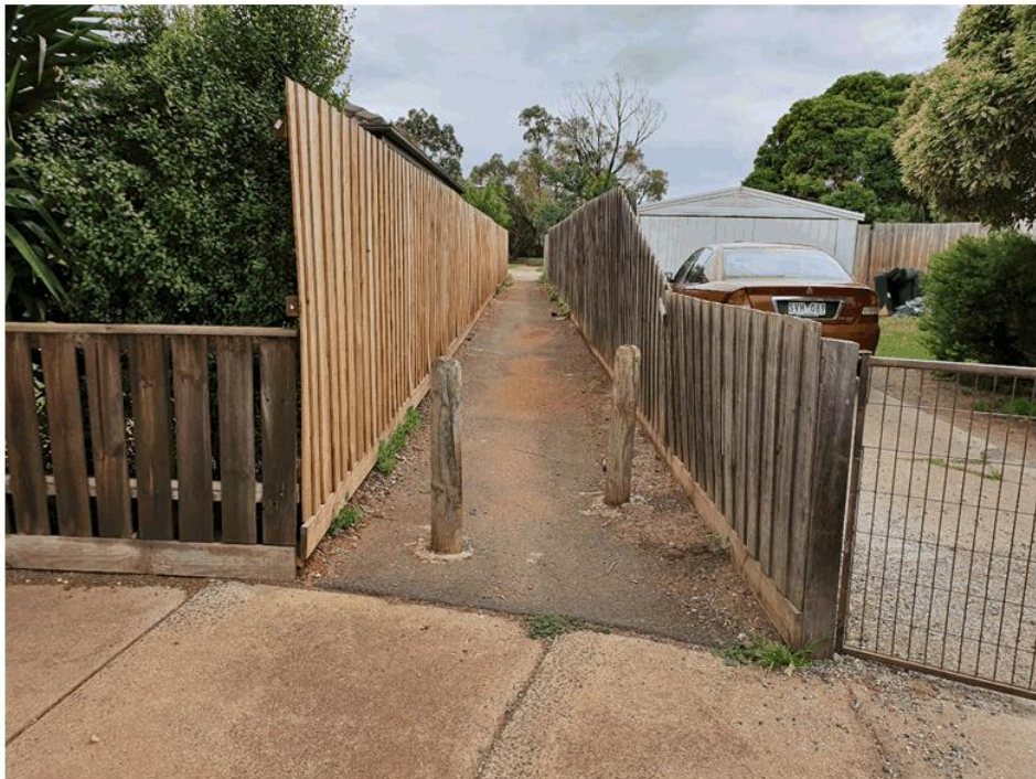
The pedestrian walkway in Vista Drive – Looking into the alleyway.
