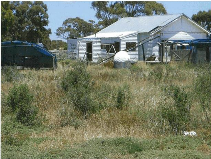
Figure 4: Dilapidated weatherboard house, view towards south
