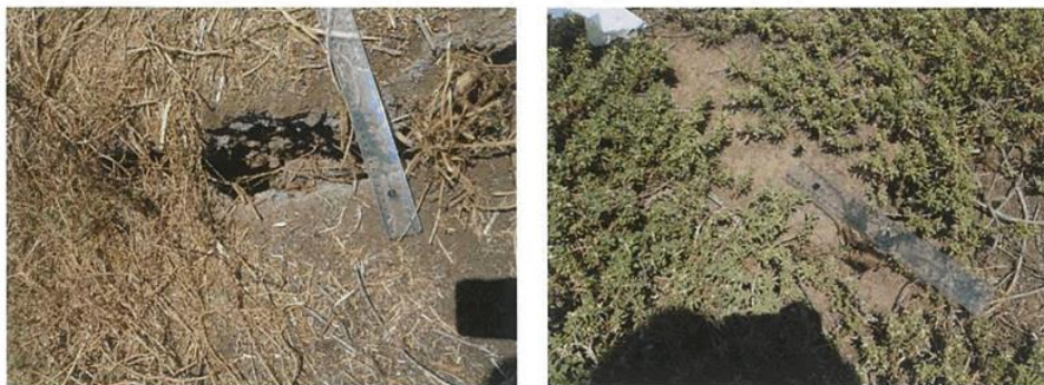
Figure 2: Examples of shrinkage cracks, some of which have apertures greater than 100 mm
