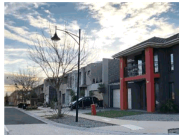
IMAGE 11: EXAMPLE OF "TERRACE HOME" DESIGN ALONG TATTERSON WAY WITHIN THE CYPRESS VIEWS (EAST) RESIDENTIAL PRECINCT
