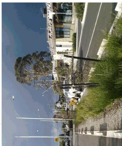
Image 30 Example of central swales allowing for water to be filtered and cleaned, prior to entering the stormwater system
