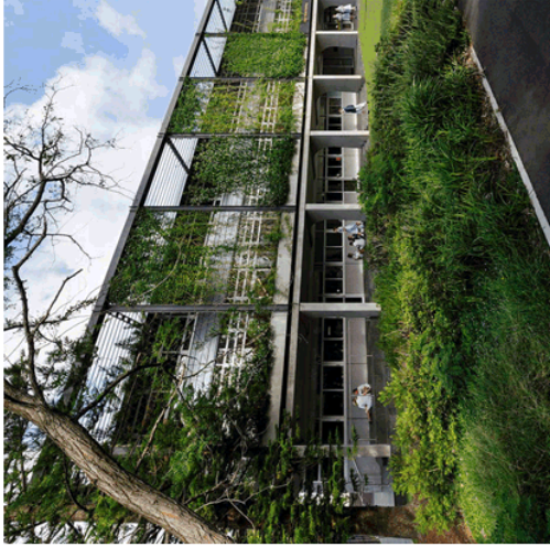
Image 27 Example of increased vegetation cover on building facades which will lower the ambient temperature of the centre
