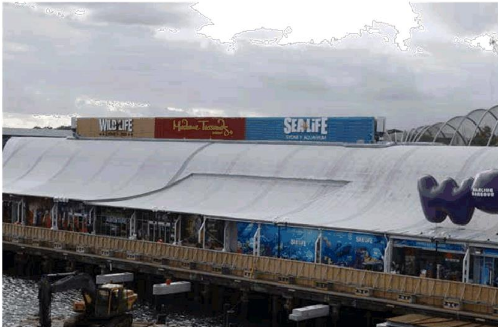
Figure 4 - A rooftop installation that does not break the ridge or overall height of the building.
