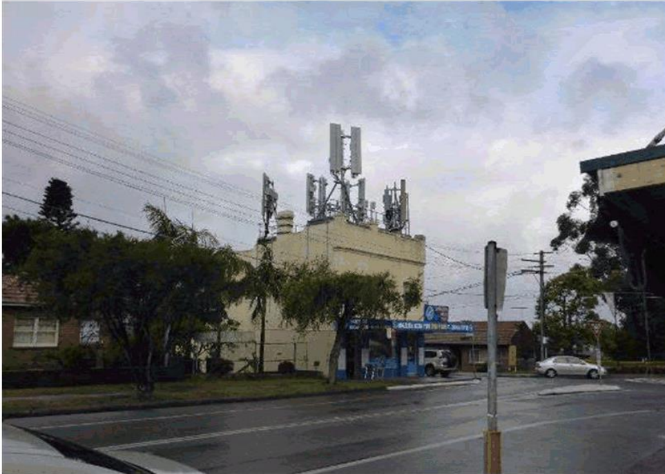
Figure 6 - An obtrusive and overcrowded rooftop.
