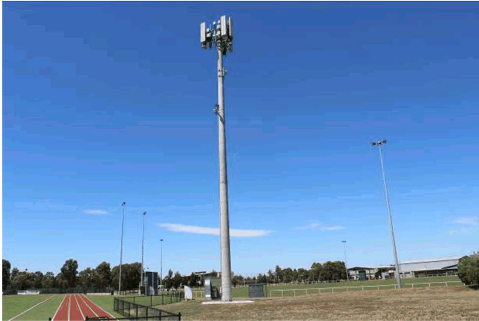
Figure 8 - A poor example of a telecommunications facility in a reserve.
