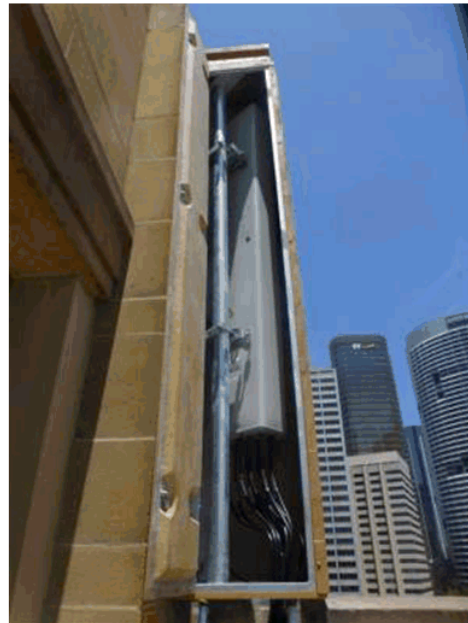
Figure 3 - An example of shrouding/screening on a prominent heritage building.
