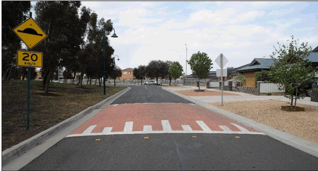
Figure 9 Flat Top Road Hump LATM Treatment
